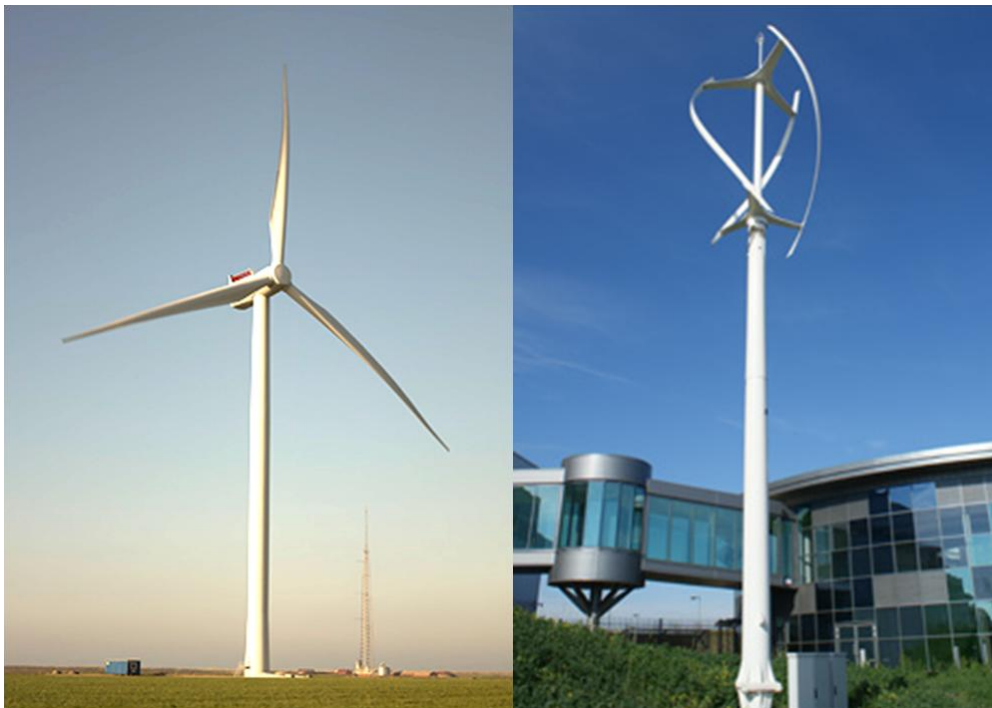
Figure 2 - Left: Large-scale HAWT Siemens SWT-6.0MW-154m [ www.siemens.com ]; Right: Small-scale VAWT in Environment Energy Centre, Leyland, UK [ www.quietrevolution.com ]
